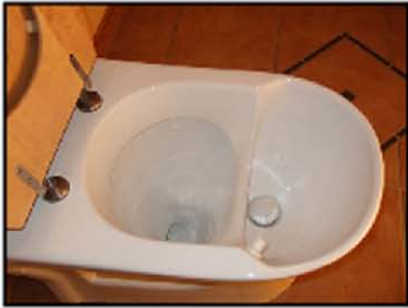
Two Swedish Urine Separating Toilets (EcoSan and Novaquatis)
